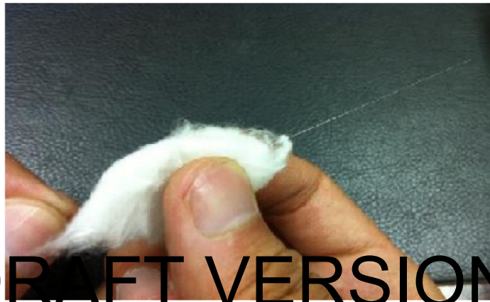
Figure 7: Cleaning the stripped fibre
