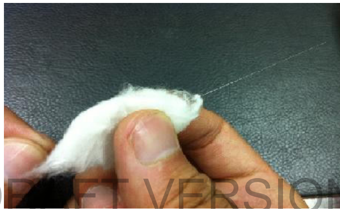
Figure 7: Cleaning the stripped fiber
